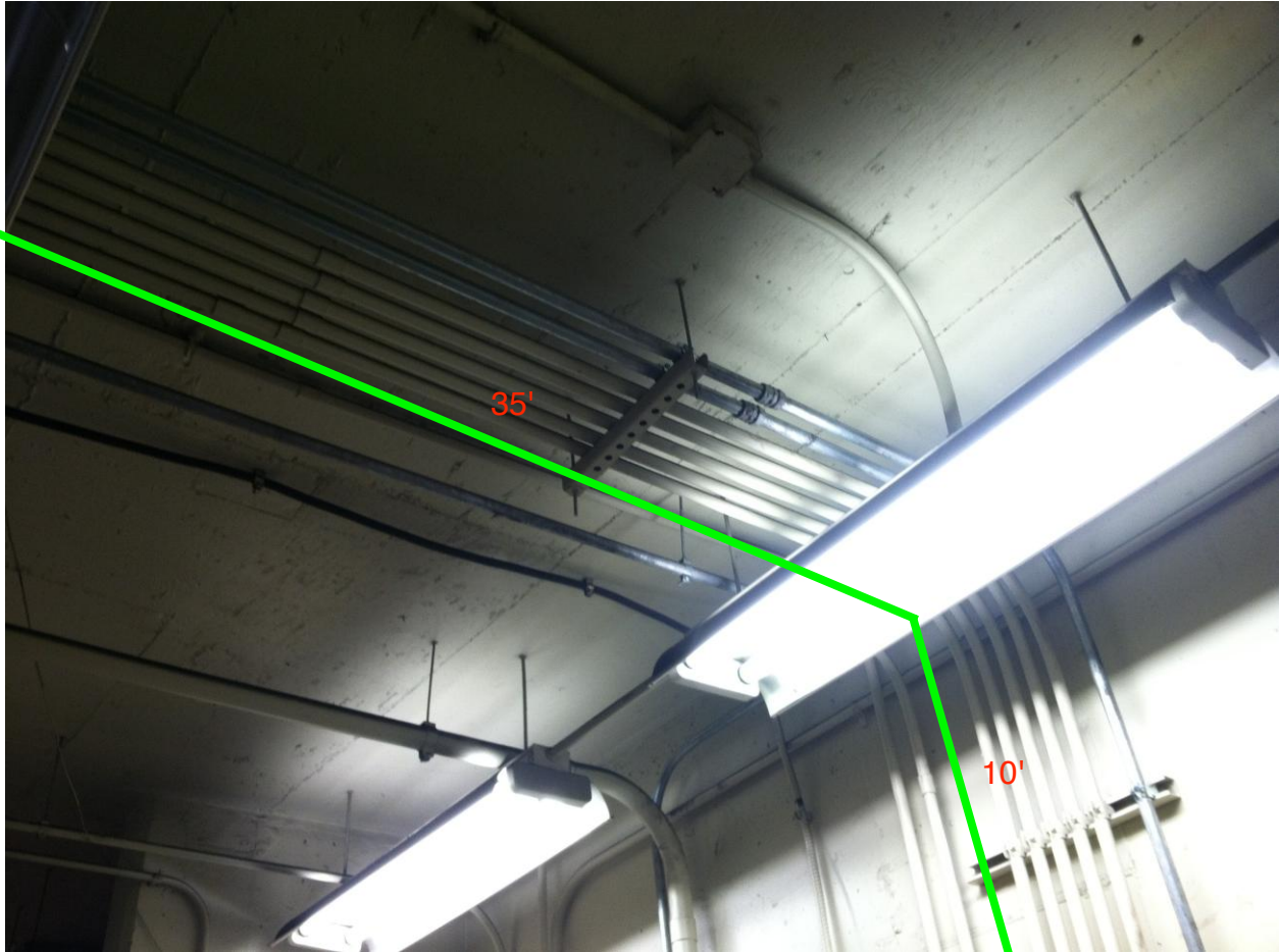
Photo 10 – Proposed overhead conduit in Room 206.
